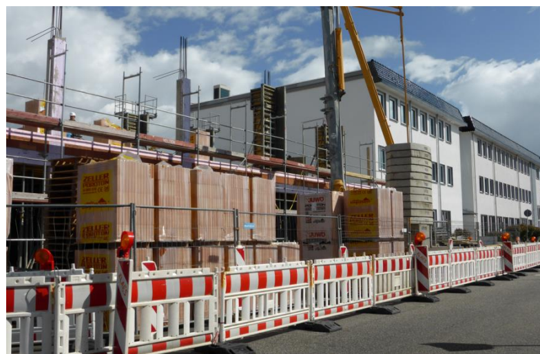
Construction site at the Giessen location
